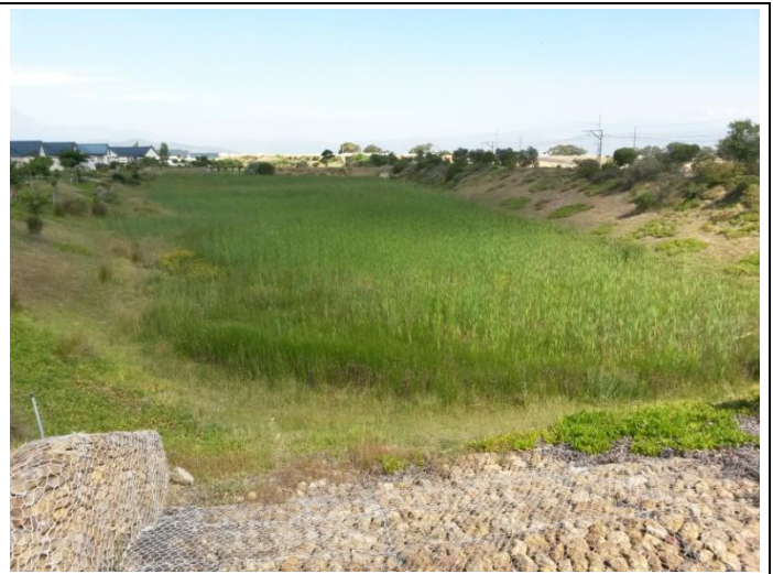
Photo 20: Another of the retention dams, containing bulrushes that were cut recently, and have subsequently begun to re-grow.
