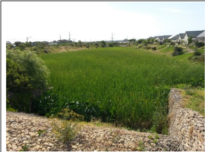
Photo 19: One of the retention ponds, stocked with fully grown bulrushes.
